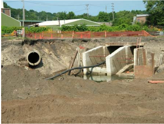
Twin Box Culvert
