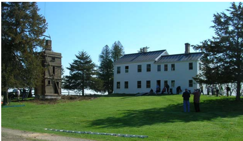
Tower's New Home
