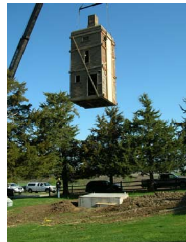
Tower Lifted to New Foundation
