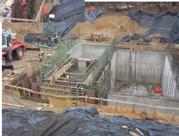
Lower Level Foundation Walls
