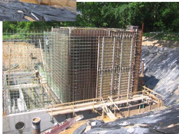
Upper Level Foundation Walls
