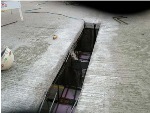
Removed Deteriorated Construction
