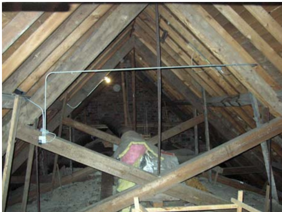
Existing Roof Truss
