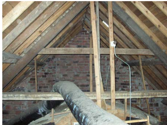
Existing Roof Frame
