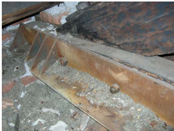
Supplemental Steel Angle with Stiffener Plates at Bearing
